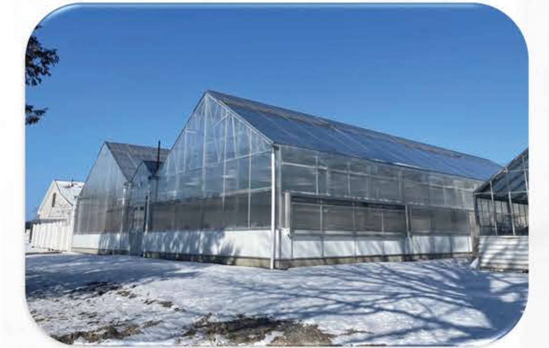
2022 Exterior of new greenhouse addition
